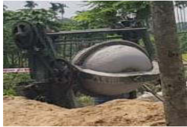
No guard in rotating armor of mixture machine reported at zone -12
