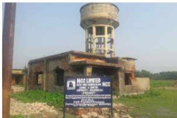
Project display board noted at Amta(Zone 1) Reservoir site. Contact numbers are missing. Urgently required demolition of old reservoir
