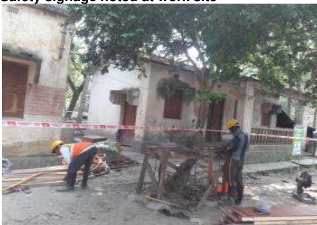
Partial use of PPEs by workers – noted. No use of hand gloves during bar bending work
