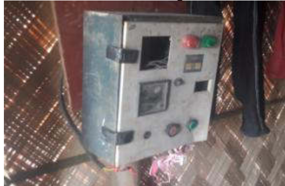
Electrical safety norms need to be maintained. Use of rubber mat below switch board is necessary
