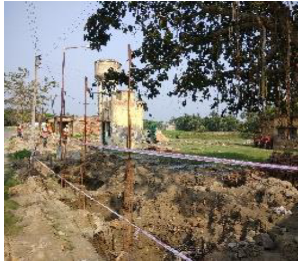
Improper storage of excavated soil from construction site seen during visit at zone-1
