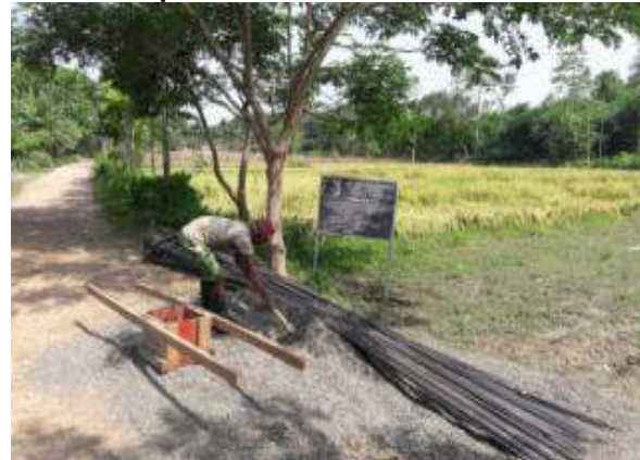
Baniyara - Zone 13 water reservoir site. Incomplete display board. No start – end date, contact no. etc. Partial use of PPEs by workers
