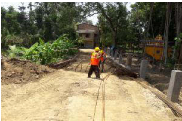
Partial use of PPEs by workers. No use of hand gloves during bar bending work
